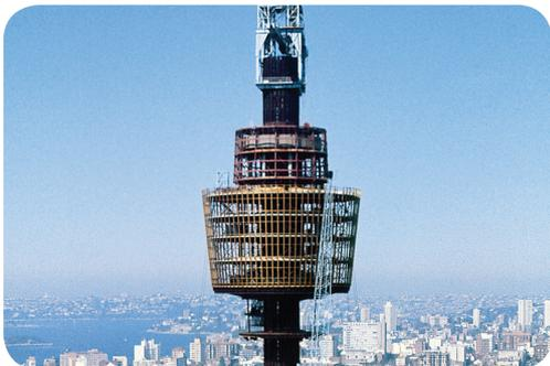
Each barrel unit was completed with lift rails, stairwells and hydraulic risers before hoisting. The shaft contains two sets of fire stairs, fire, electrical and plumbing ducts in one half and the lift shafts in the remainder.
