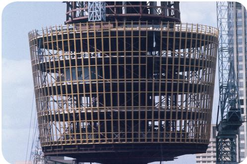
Pre-made individual barrel units formed the shaft of the tower and the four levels of the turret structure were constructed at the base of the shaft and raised to the top as work progressed.
